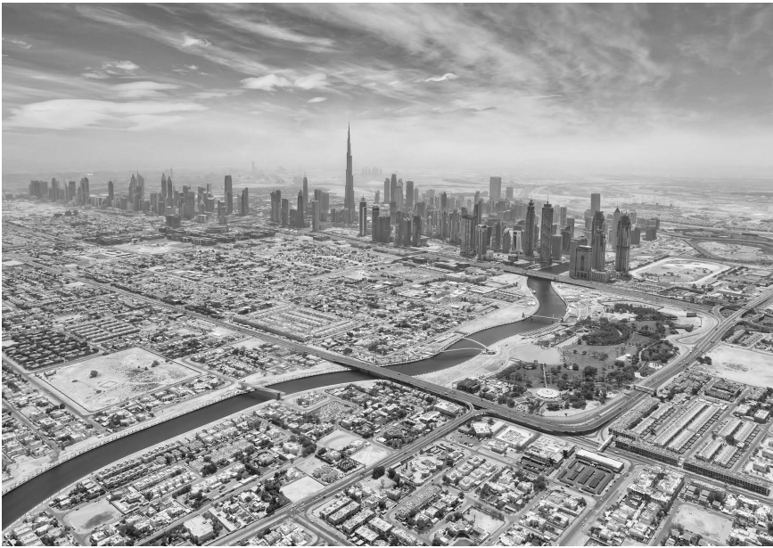
Figure 4.6 Dubai Water Canal, a transformative project for the city.
